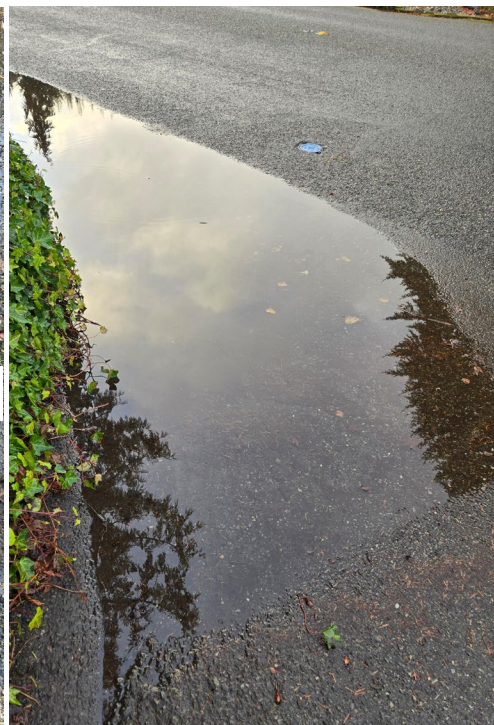
Results of a Blocked Stormwater Drain
