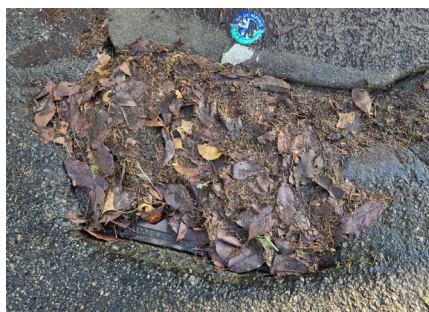
Blocked Stormwater Drain
